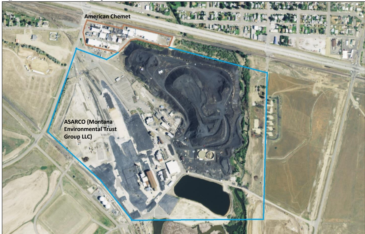
Figure 1.1 - Aerial Photograph of the American Chemet and ASARCO Facilities before Demolition
